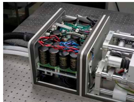
Power supply for pump diodes located inside laser head
